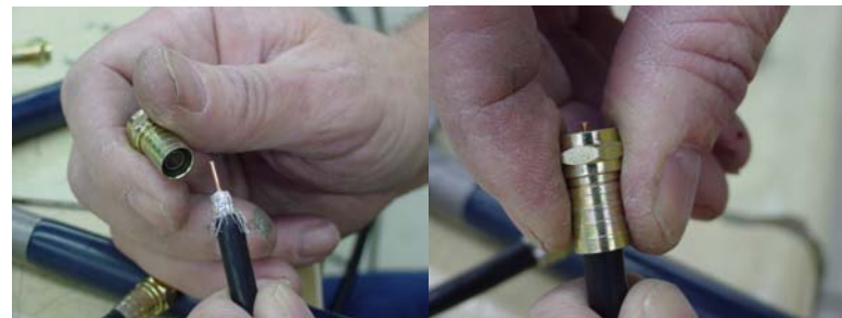
Attach Coax Connector to end of Coax Cable
