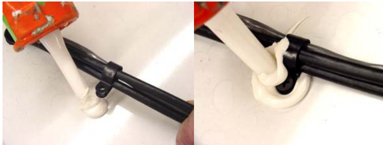
Put a dab of Dicor under a plastic cable clamp before you drill a hole to secure the clamp. After it is screwed in, cover the rest of the screw with Dicor.
