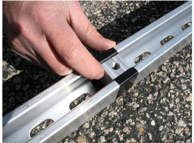
Step 4 – Place one of the rails on the ground and slide the two T-nuts into place on the two black marks.
