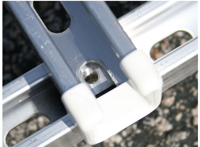
Step 5 – Place the other rails together as shown. Line up the top rails so that ends are above the T-nuts.
