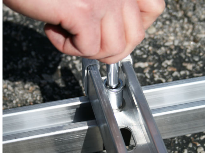
Step 7 - A ratchet wrench and a 9/16 socket is used to secure the four bolts on the rails.
