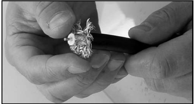
Figure 87: Flaring the Braid
