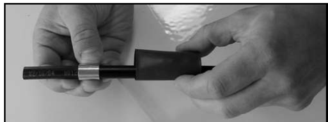
Figure 81: Placing the Heat Shrink Tubing and Ferrule
