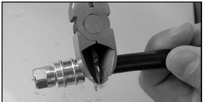
Figure 108: Trimming the Braid
