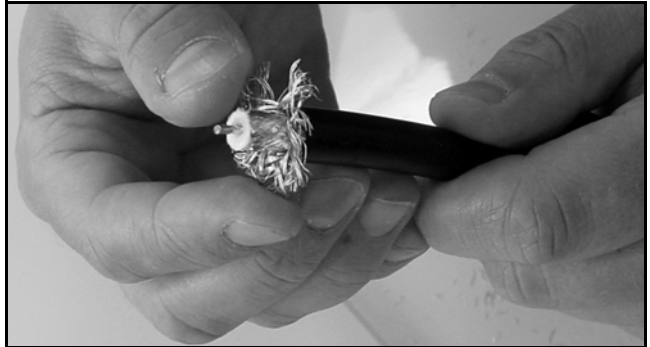
Figure 100: Flaring the Braid
